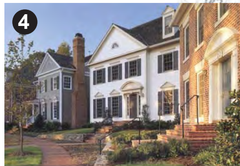
Narrow-Lot housing with garages at alleys - Kentlands, MD
